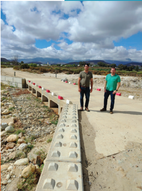
Figure 14: Mentor Nico Jonker's candidates Daniël Neethling and Marius Norman at a low-level crossing that Marius designed and rebuilt after washaway
